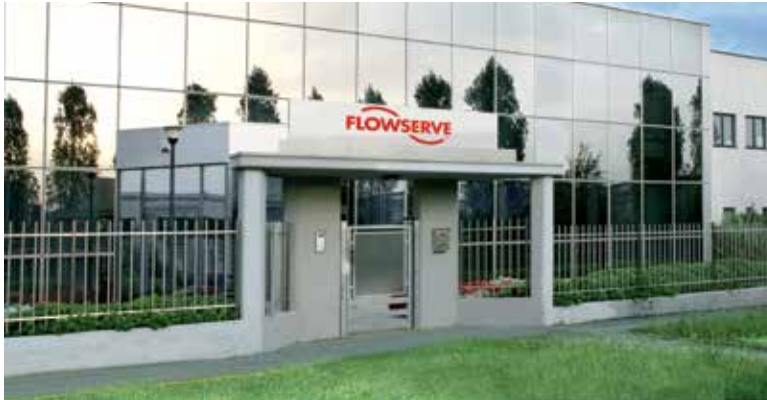
Flowserve Valbart Main Office
