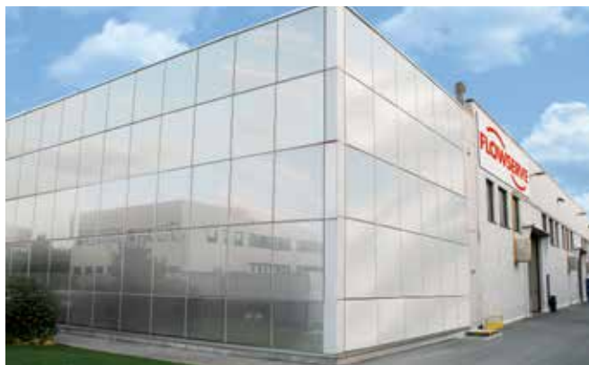
Flowserve Valbart Testing and VAC Centre
