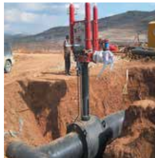
Welded body valve with extended stem
